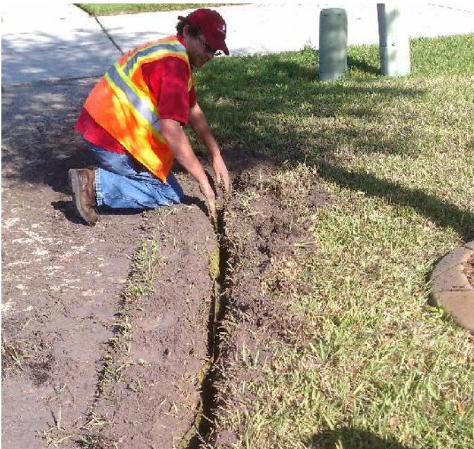
Installation of BioBarrier after root pruning
